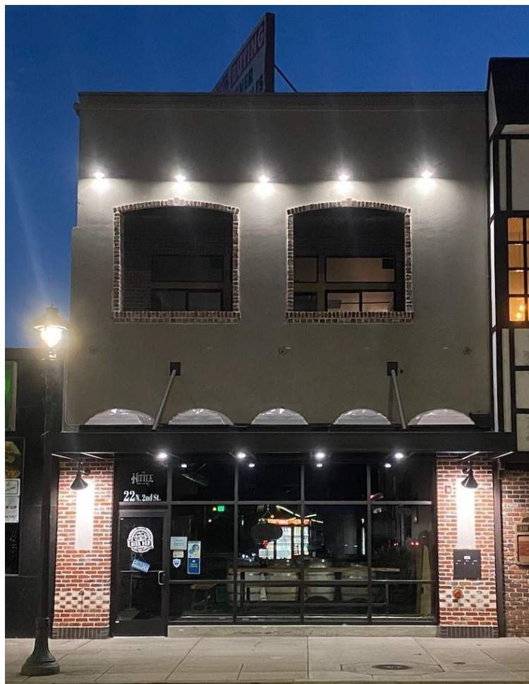
2019 Project The Hittle Building
